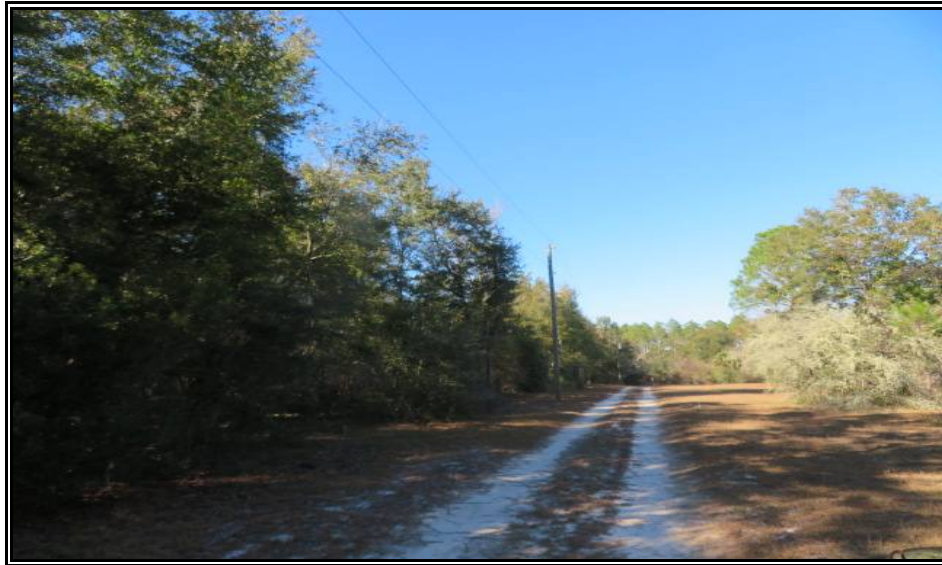
View of Access Rod/Riley Drive
